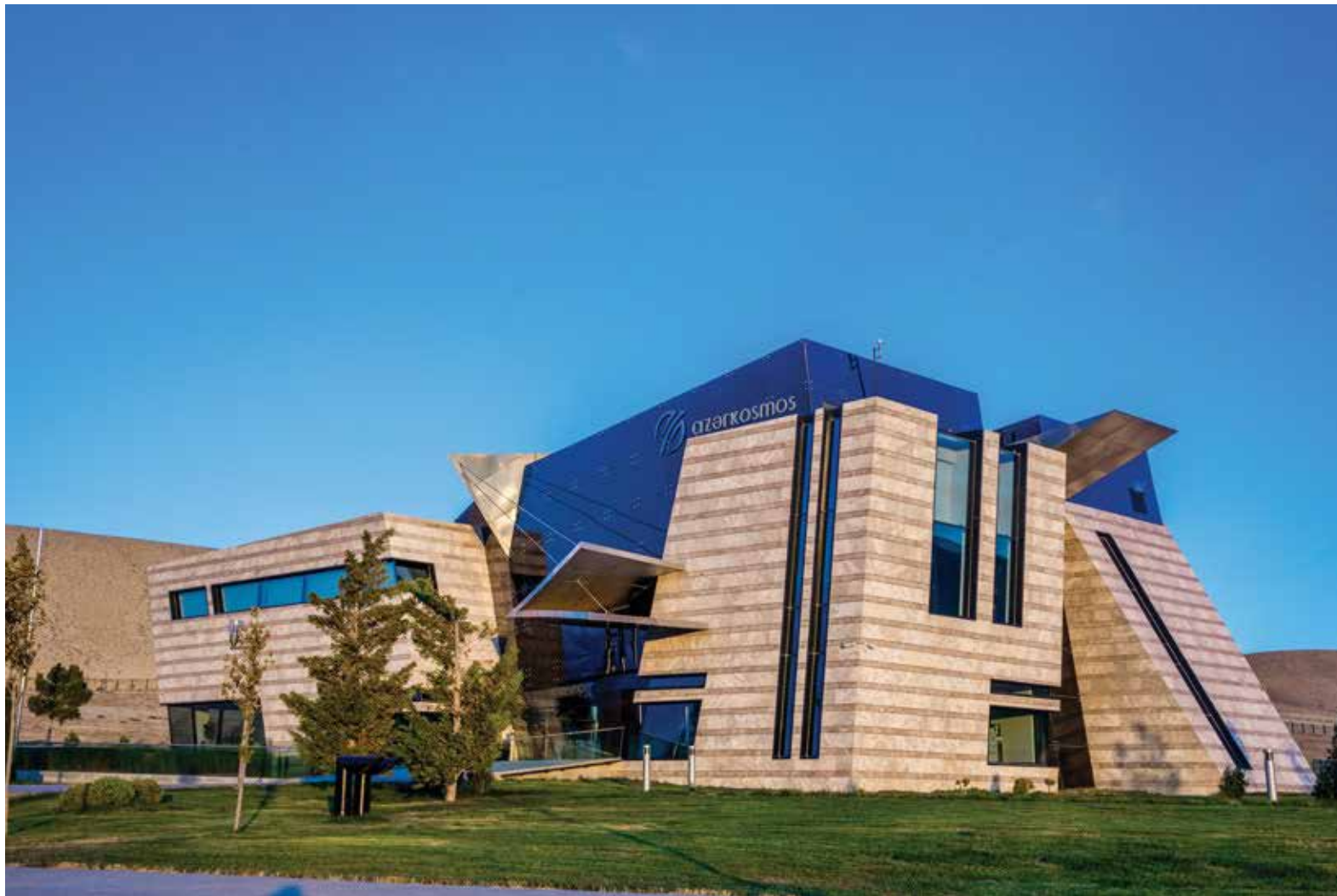
Main Satellite Ground Control Station Baku-Shamakhi Highway
