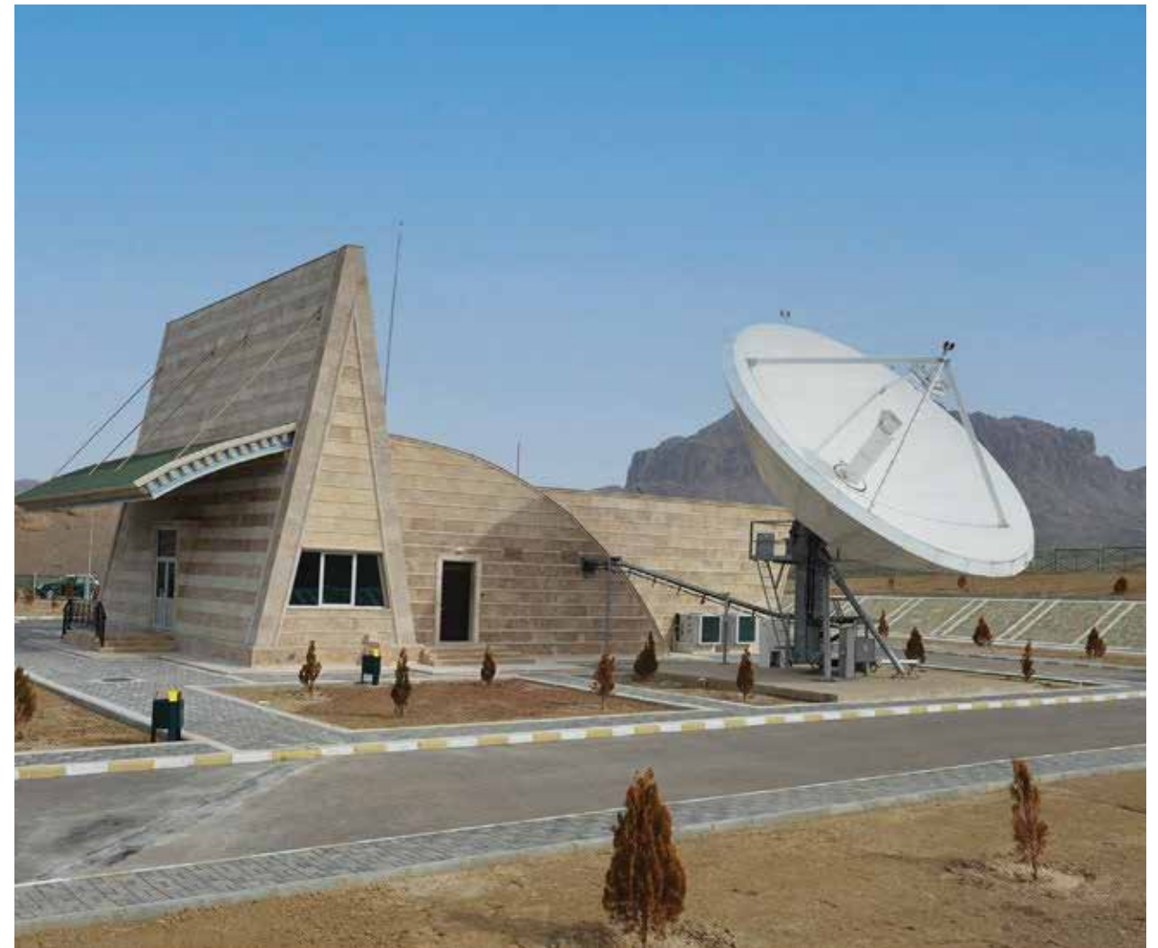
Back-up Satellite Ground Control Station Julfa region, Nakhchivan
